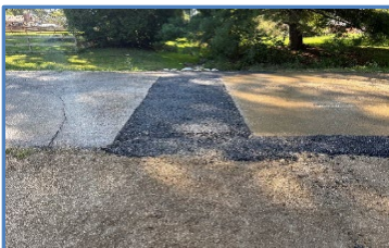
Culvert pipe replacement on Donald Dr
